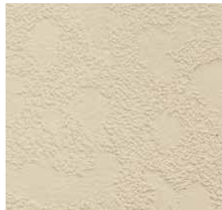
Item Plaster and Paint
